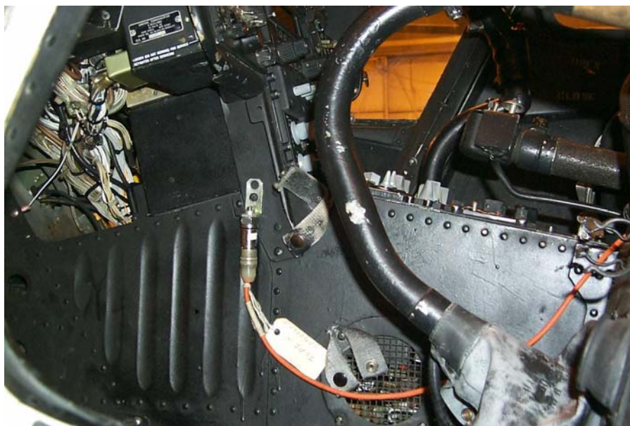
Figure 4. Vertical Accelerometer Installation
